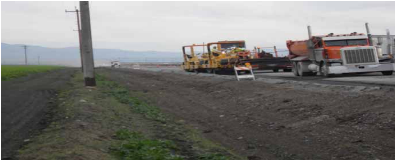
Paving on Stage 2 Shoulder
