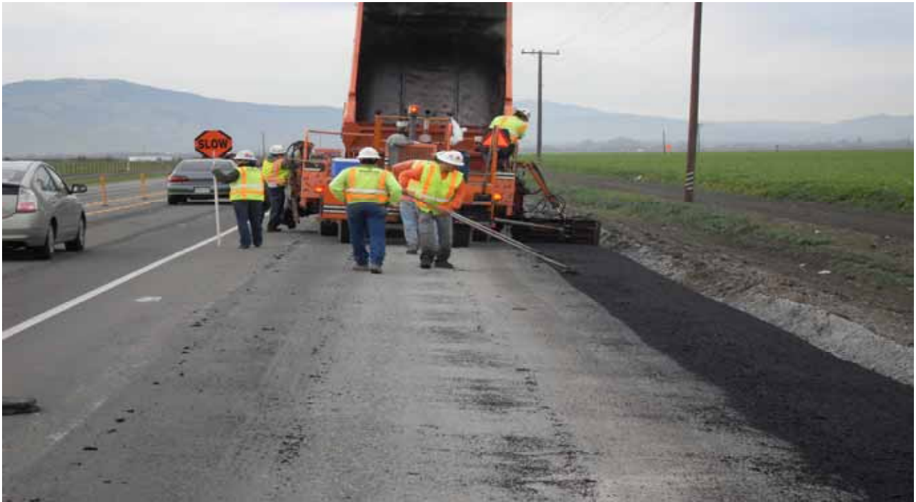
Paving on Stage 2 Shoulder
